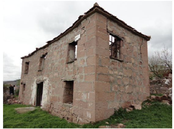
Figure 6. Examples of stone masonry buildings with inadequate load-bearing walls in each of the orthogonal directions in plan
