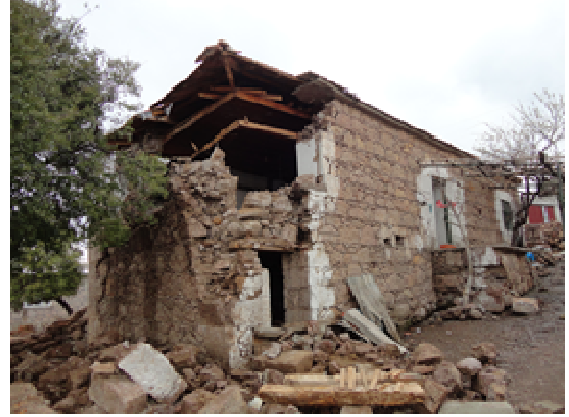
Figure 5. Examples of heavily damaged two-storey stone masonry buildings
