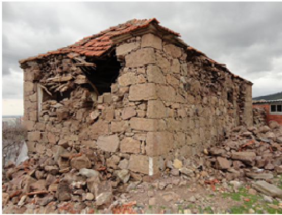
Figure 6. Examples of stone masonry buildings with inadequate load-bearing walls in each of the orthogonal directions in plan
