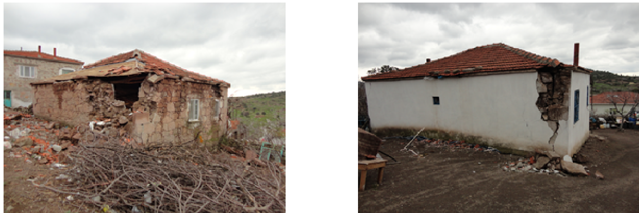
Figure 11. Examples of failure of masonry building corners
