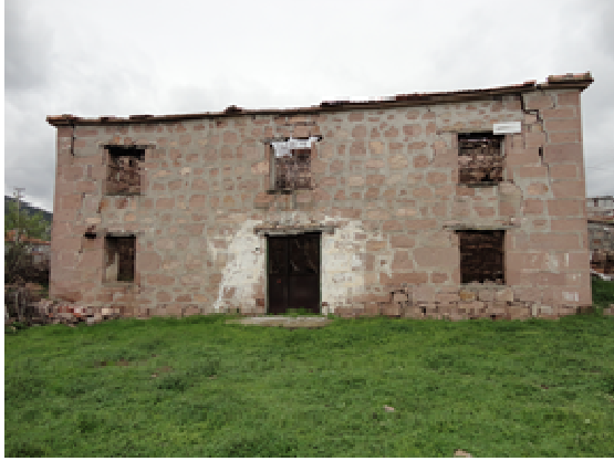
Figure 5. Examples of heavily damaged two-storey stone masonry buildings
