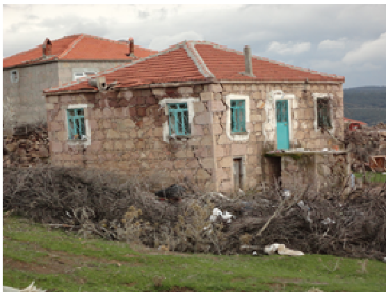
Figure 7. Examples of masonry buildings which the nearest window or door opening to the corner was less than 1.50m
