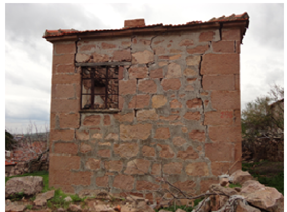
Figure 7. Examples of masonry buildings which the nearest window or door opening to the corner was less than 1.50m
