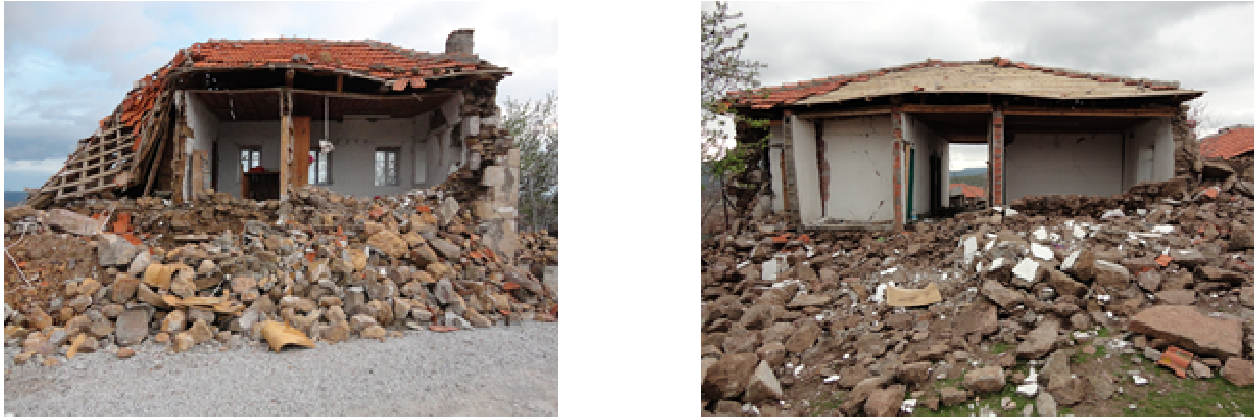
Figure 8. Examples of masonry buildings whose outer walls were stone and the inner walls were brick or wood
