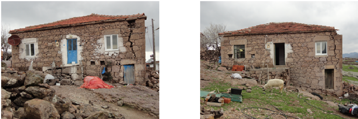
Figure 9. Examples of masonry buildings with partial basements
