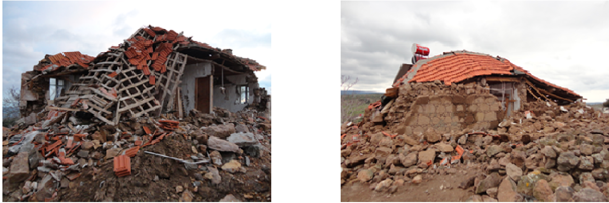
Figure 3. Examples of completely collapsed masonry buildings
